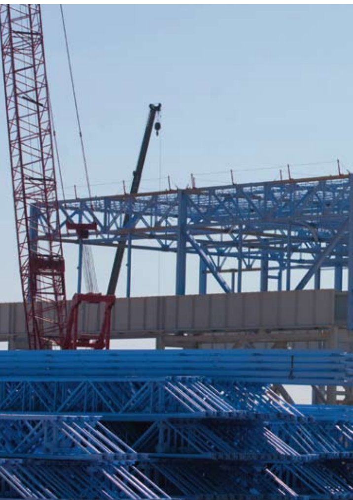
ThyssenKrupp Steel USA Hot Strip Mill under construction
