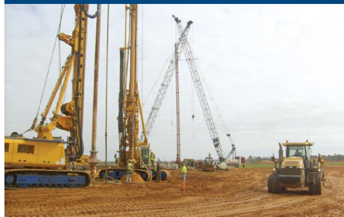
A steel column is erected on site as building construction begins.
